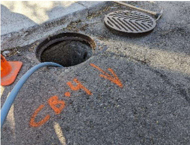
9. CB-4 and CB-5 on Campbell connect to COMB-C (green dye)
