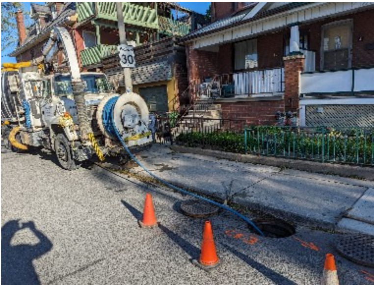
5. CB-3 Ernest connect to COMB-B (green dye)
