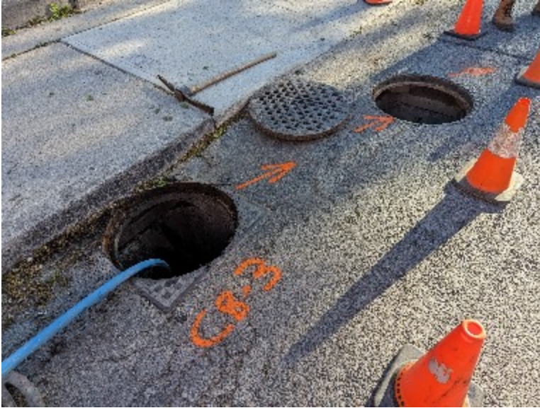
6. CB-3 Ernest connect to COMB-B (green dye)
